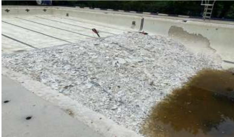
Using chipping guns, chip off all old pool plaster (currently there are 6 layers of plaster on the pool.)
