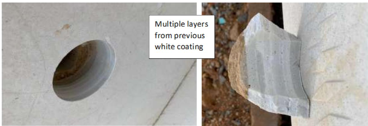
**What's Involved:** Chip out and remove pool plaster down to the gunite (see picture below)
